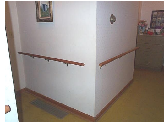
Stair rails make an attractive grab bar - or exercise bar - in this home.
